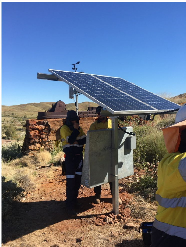
Permanent blast monitoring station at Klondyke Queen
